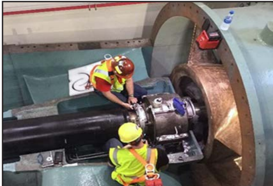
Refurbishing water remediation pump.
